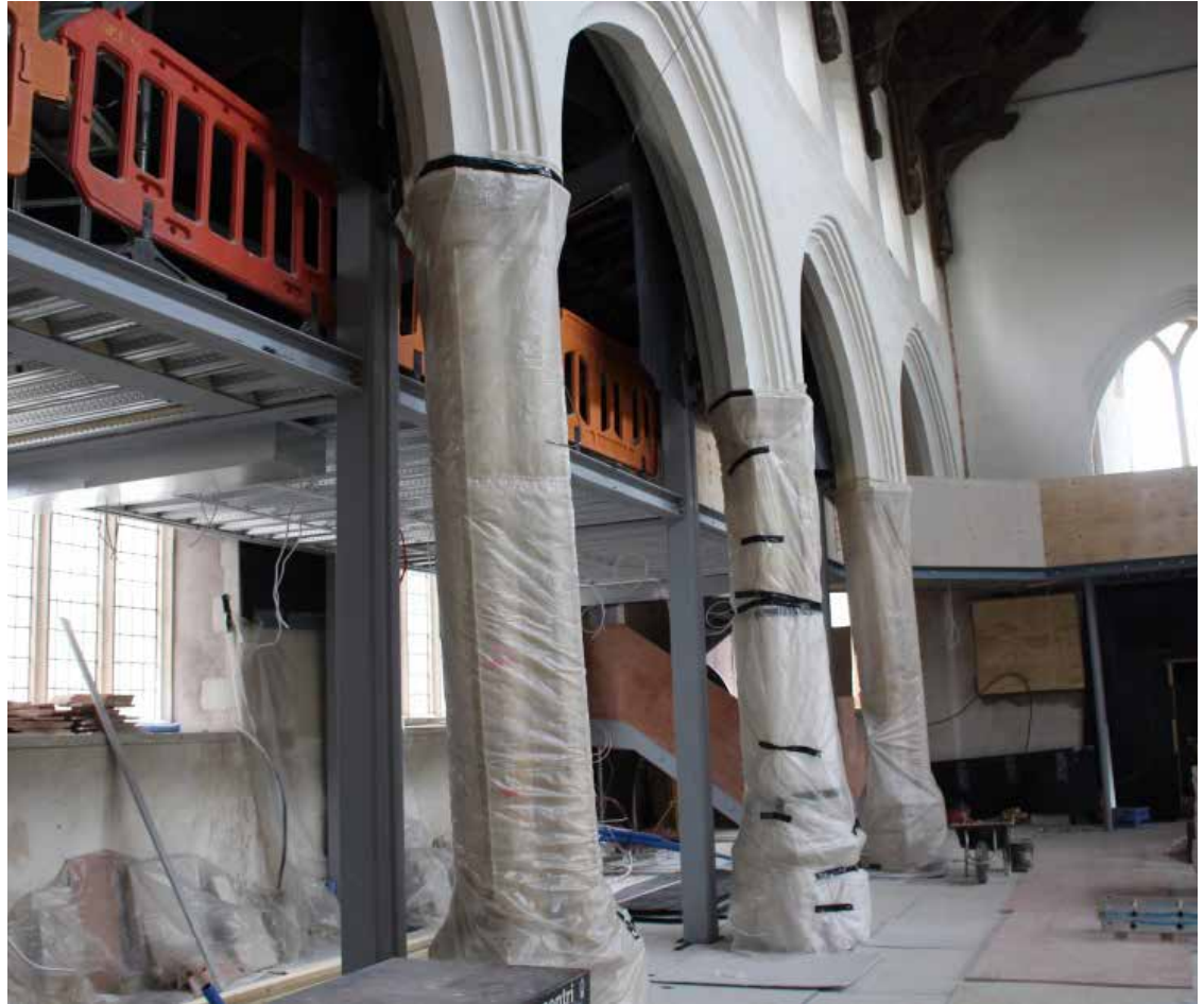
Fig. 9 The new mezzanine provides structural support as well as meeting space
