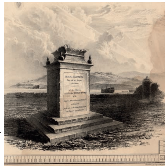
Fig. 5. Deterioration of the first monument built to John Moore in 1811. Drawing by Captain William Willermin (Wyld, Maps and Plans... )
