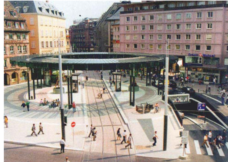
Figures 8 & 9 -Square Homme de Fer before and after the renewal Images by architect
