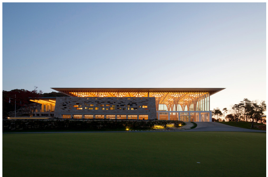
Figure 2: External view of the Nine Bridges Country Club designed by Shigeru Ban. From this picture emerges the structural system based on a regular layout of timber columns that support the big roof and strongly define the internal spaces.
