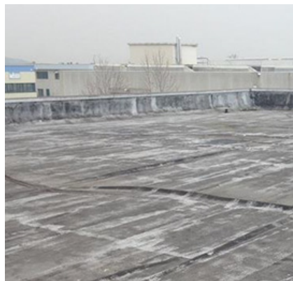
Figure 1: Old damaged sheath
