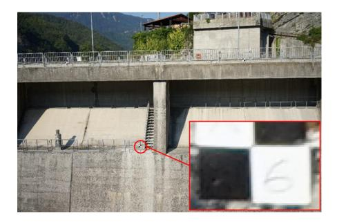
Figure 2: Frame of the downstream face, taken from 30m distance, in which, performing the maximum zoom, the number and the centre of the marker are perfectly detecteble
