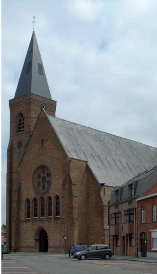
Fig. 6a Church of Our Lady, Poelkapelle. Project “New Life @ Church” on partitioned use. Example of a typical large interbellum church of the Westhoek, Poelkapelle (photo https://inventaris.onroerendergoed.be )
