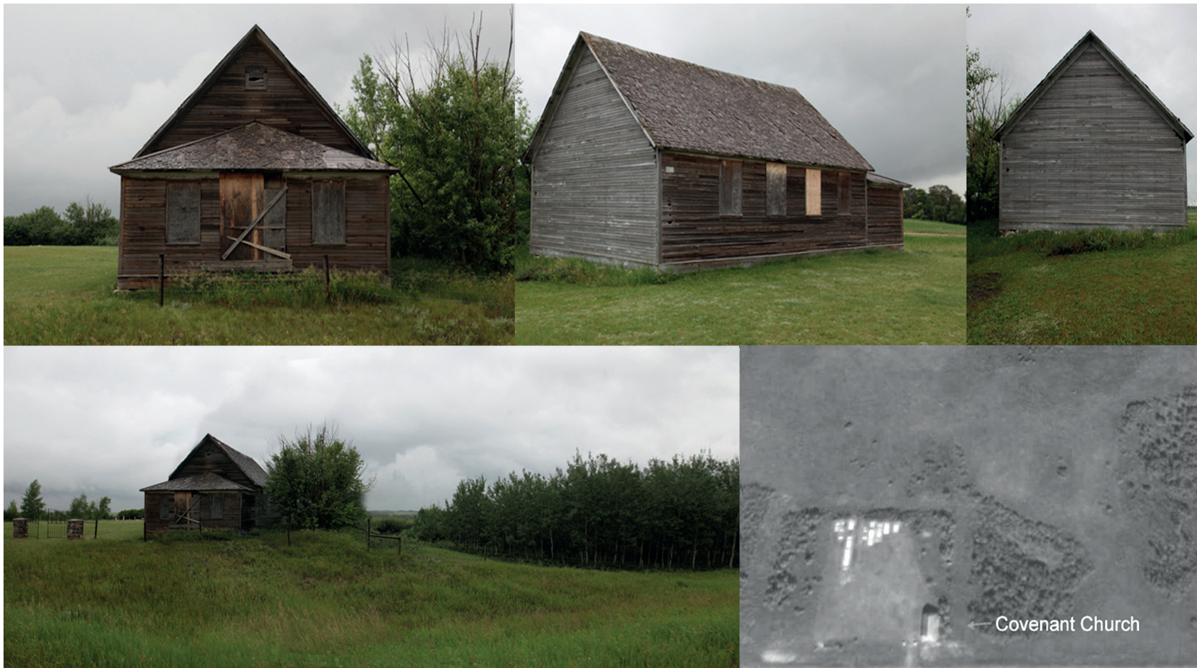
Fig.1 Covenant Church, northeast of Young, Saskatchewan, Canada, built in 1916 (photograph by author)
