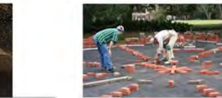
A father and son masonry team were on site to guide others in the demolition of the previous wall and then re-use the salvaged bricks to create a distinct patio that is built in the old footprint.
